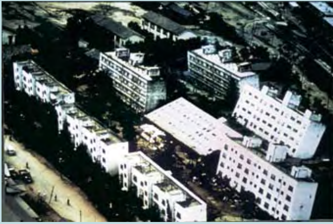
Liquefaction caused these apartment buildings to tip over during the 1964 magnitude 7.4 Niigata, Japan, earthquake (Earthquake Engineering Research Institute.)
