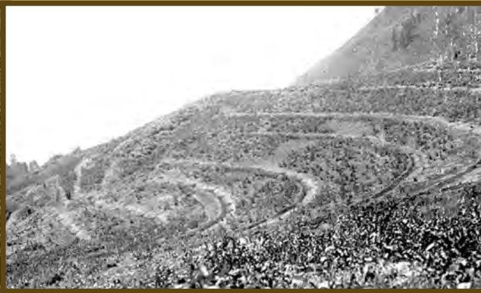
Laborers from the CCC Hobble Creek Camp constructing erosion-control terraces (left) and completed terraces (right). Location unknown but presumably in Utah County near Springville and the Hobble Creek drainage basin. Photos courtesy of the Utah Historical Society.
