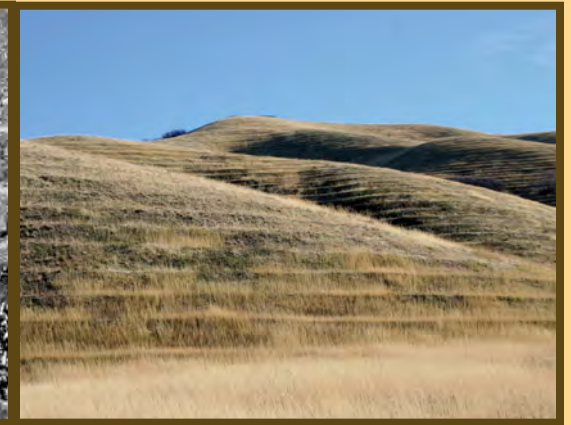
Recent photo of erosion-control terraces constructed by the CCC in the 1930s, above the Bonneville shoreline in North Salt Lake, Davis County.
