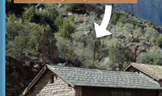
Rock-fall protection fence installed in Zion National Park to protect a maintenance building that has been struck by multiple rock falls.
