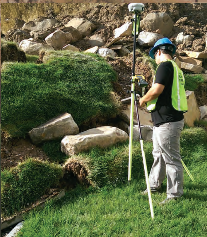
UGS engineering geologist monitoring movement of the Parkway Drive landslide with GPS equipment (photo courtesy of Ben Erickson).
