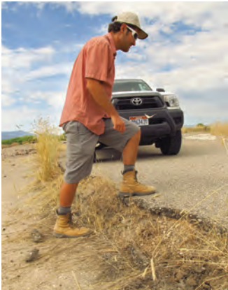
UGS geologist Tyler Knudsen examines roadway damage from a subsidence-related earth fissure in a partially developed residential subdivision in northern Cedar Valley, Utah. Photo date: July 2, 2015.
