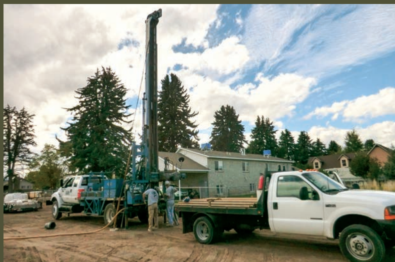
UGS oversees drilling on one of four new monitoring wells in Monroe City.
