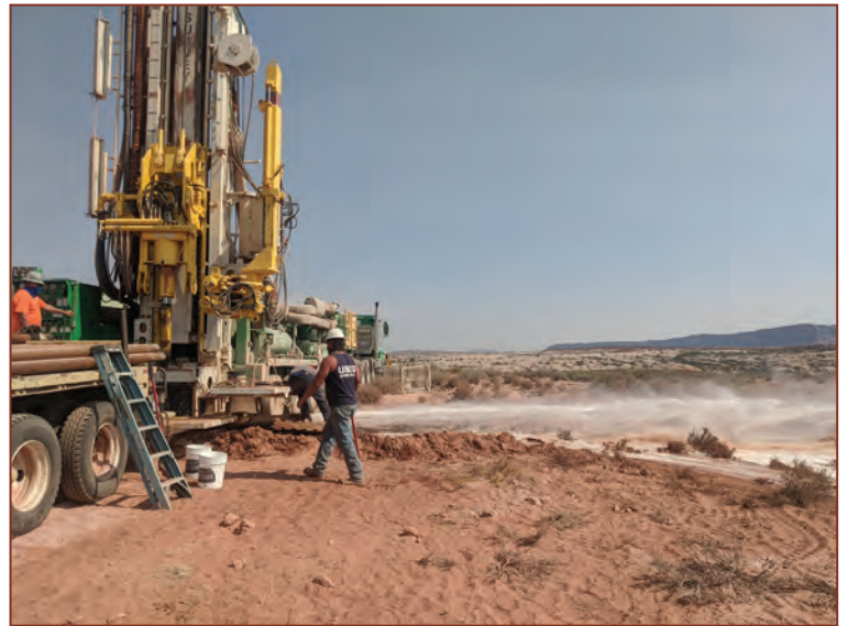
Groundwater discharge while drilling in the Navajo aquifer.
