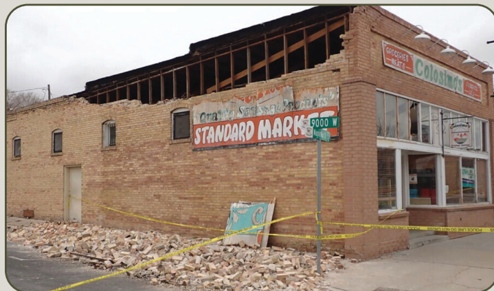
Structural damage to an unreinforced masonry building in downtown Magna caused by strong ground shaking from the Magna earthquake. Utah Geological Survey photo.
