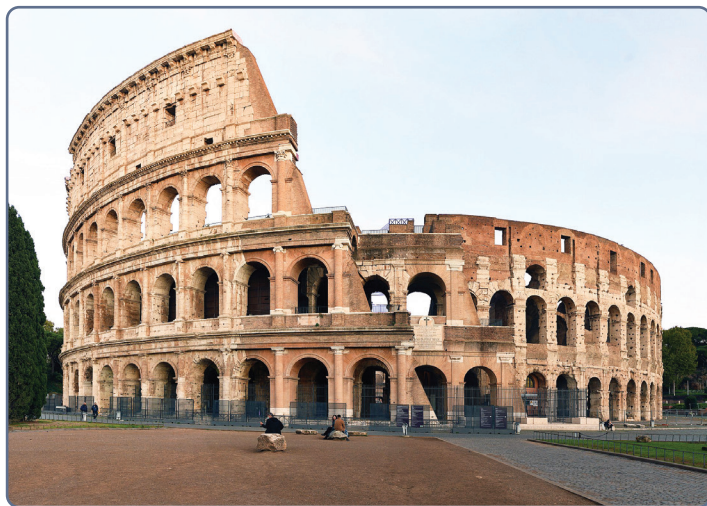
The Colosseum, which utilized pozzolanic materials in its concrete, still stands today, nearly 2,000 years after construction.
