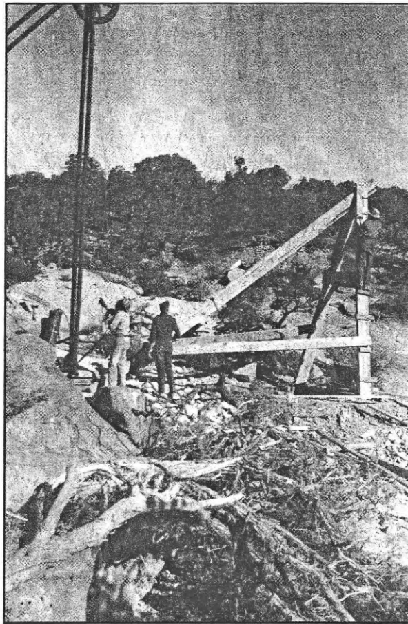
This was one of the first pictures taken at the head frame at the new Mi Vida mine, 1953.
