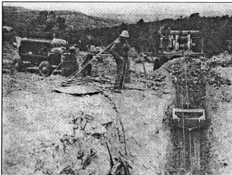
Slushing operation at the Yellow Circle Mine.
