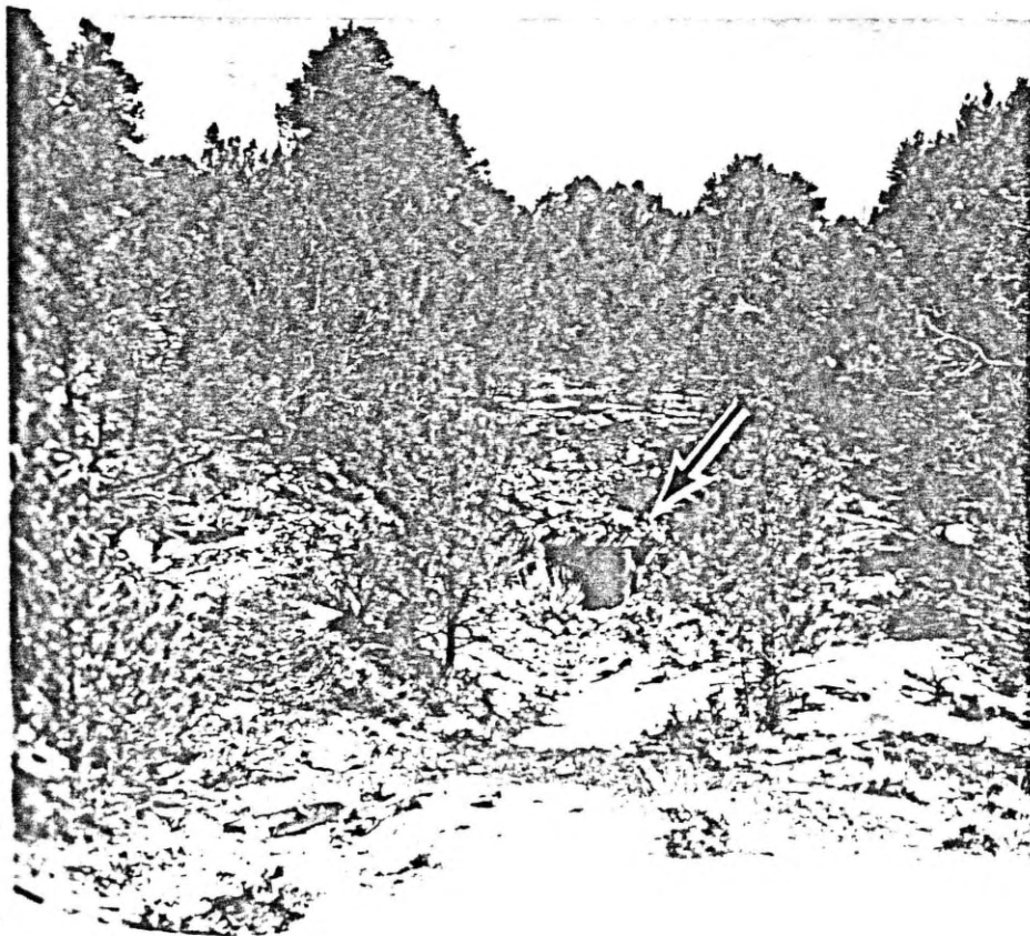
Figure 6. Independence adit. Arrow indicates the partly caved in portal as seen from the dump, looking northeast.
