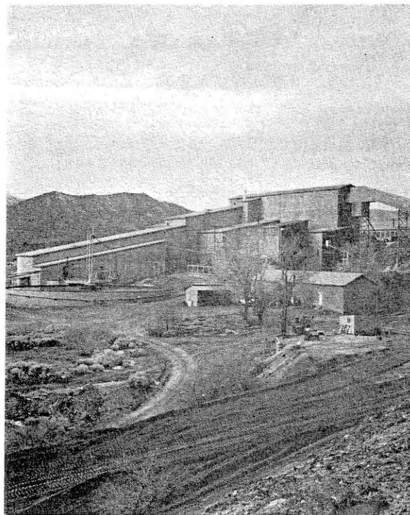
CASELTON MILL can process 1,500 tpd of mine run ore through three grinding circuits and two differential flotation lines.
